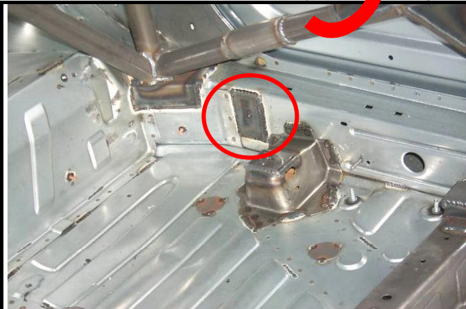
Photo des fixations des harnais/Photo of safety harness mounting
